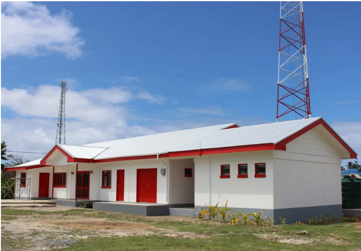
New Multipurpose Training Center for Tonga Red Cross Society in Ha'apai, funded under Japan's GGP.
